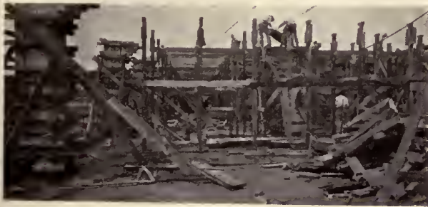
FIG. 2. SHOWING METHOD OF ERECTING SUPPORTS
